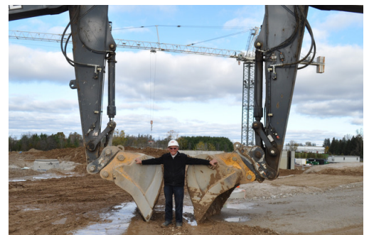
Jim Keating on the New Groves Hospital Site
