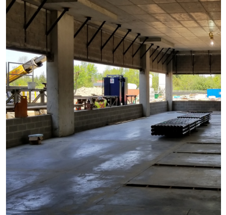
Level 1 view of Concrete structure
