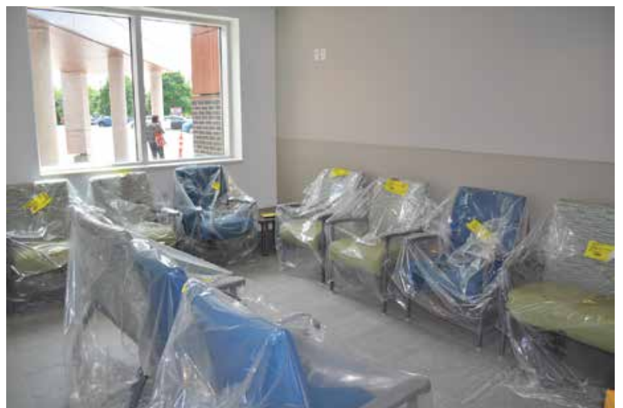
New emergency room waiting area – furniture has arrived.
