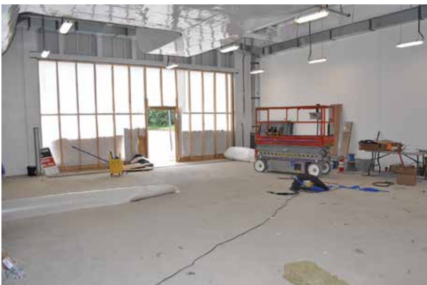
New covered ambulance garage that accommodates two vehicles.
