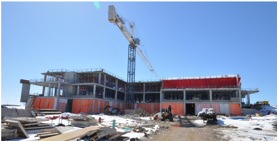
New Groves Hospital Construction – April 2018
