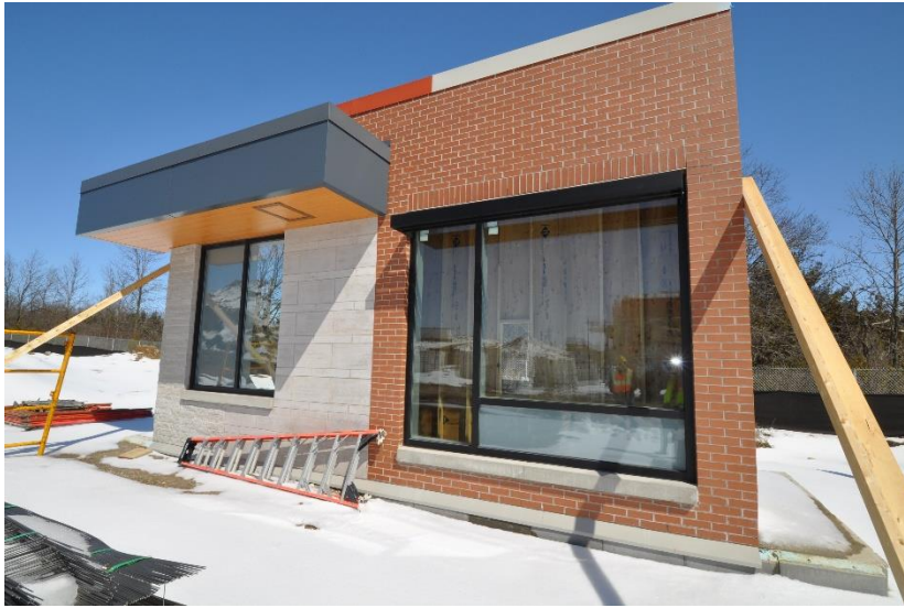
New Groves Hospital Exterior mock-up wall
